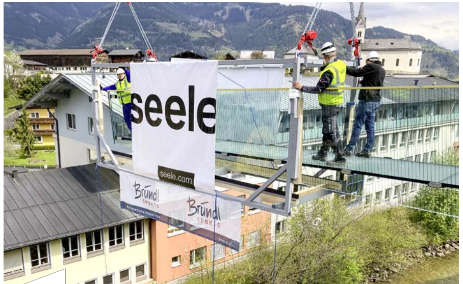
At 15 m height, seele's installation technicians dismantle the installation frame after fixing the glass walkway.
