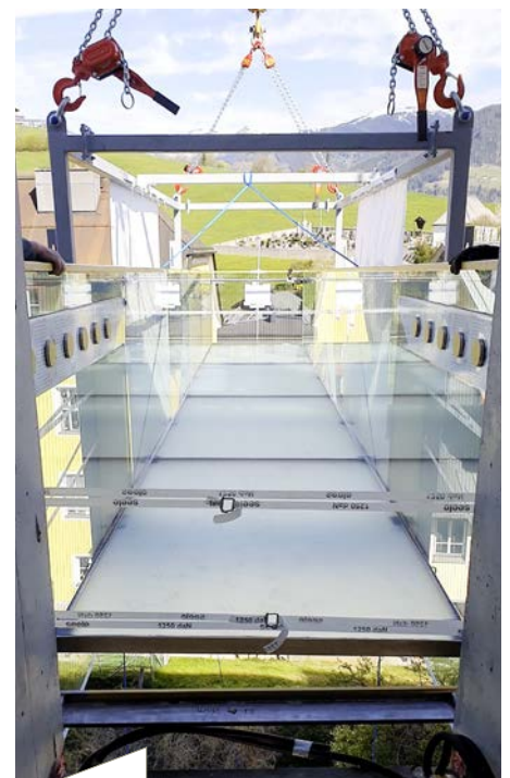
The glass walkway protrudes by 10 m from the flagship store of Bründl Sports. The special connection to the existing building allows maximum transparency
