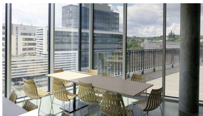
05: The eyrise glazing allows natural daylight into the interior while preventing glare and overheating when the sun is low in the sky.
