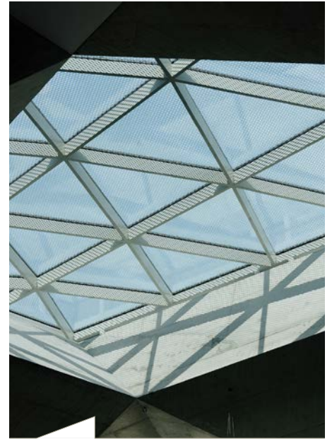
The triple insulating glass of the skylights, fitted with Okatech expanded metal, has a U-value of 0.9 W/(m 2 K) and a g-value of 21%.
