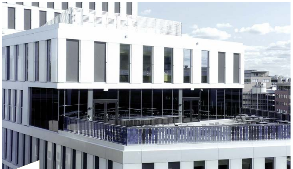
04: The 82 m 2 glass front of the cafeteria in the Orkla City complex in Oslo consists of 23 eyrise liquid crystal panes of different sizes.
