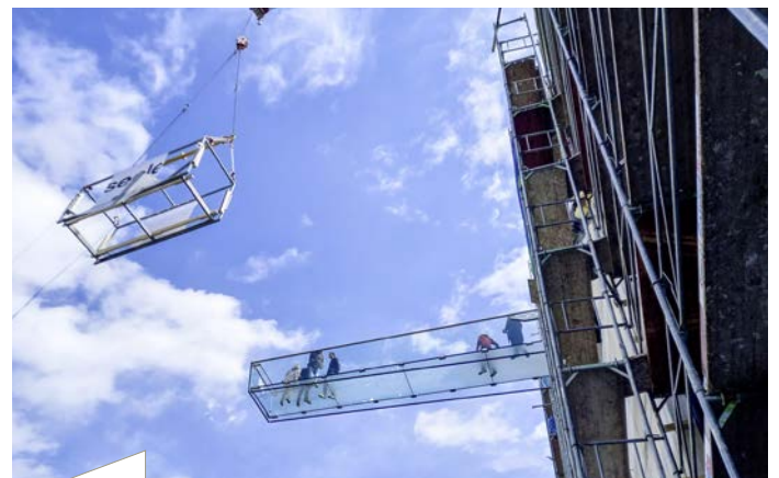
After the glass walkway was fixed to the building, the mounting frame was removed. The Skywalk rises freely from the 4th floor of the Bründl Sports flagship store.
